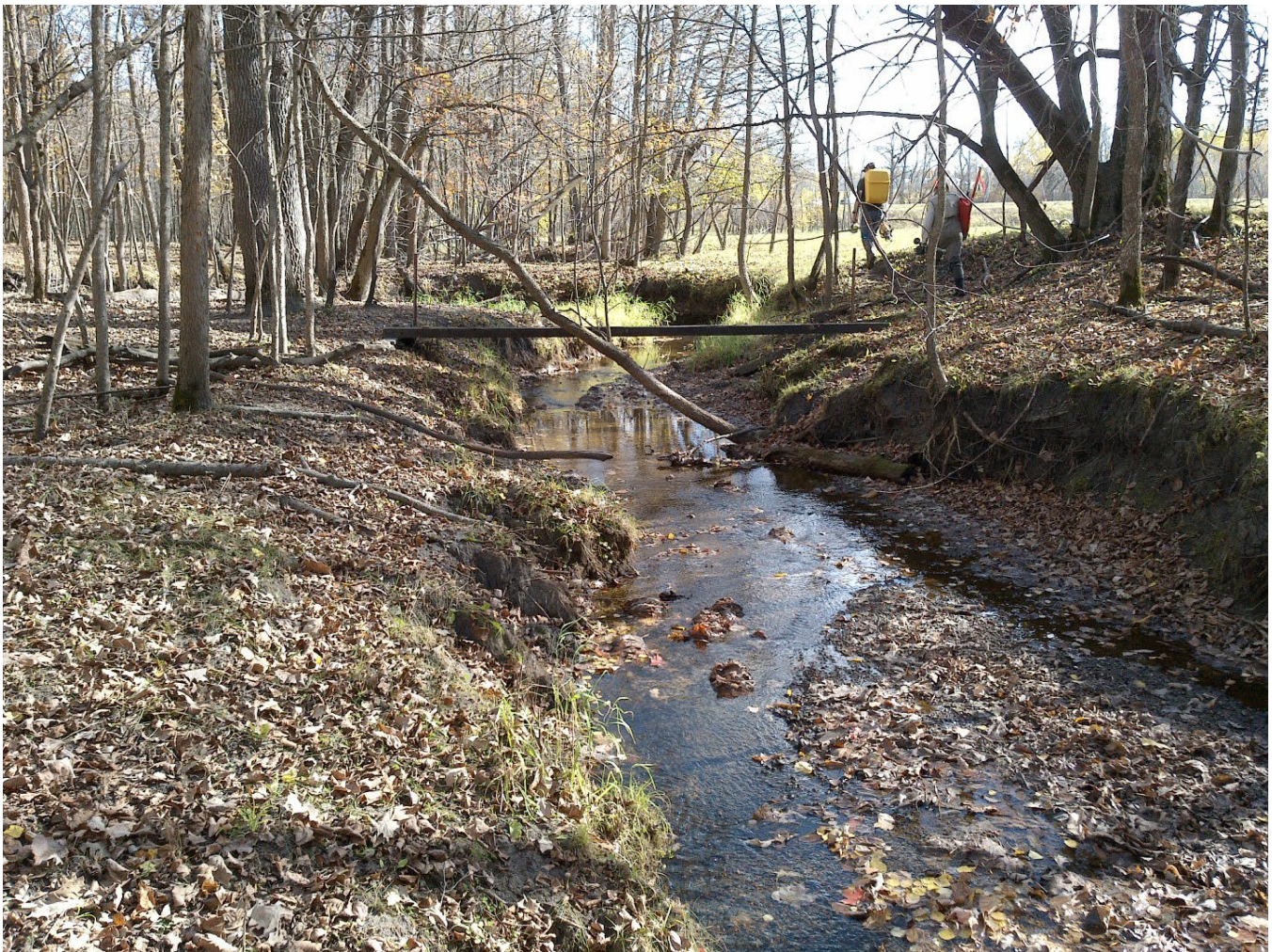
Figure 5.23. Example of bank erosion on Campbell Creek. North of CSAH 149.
