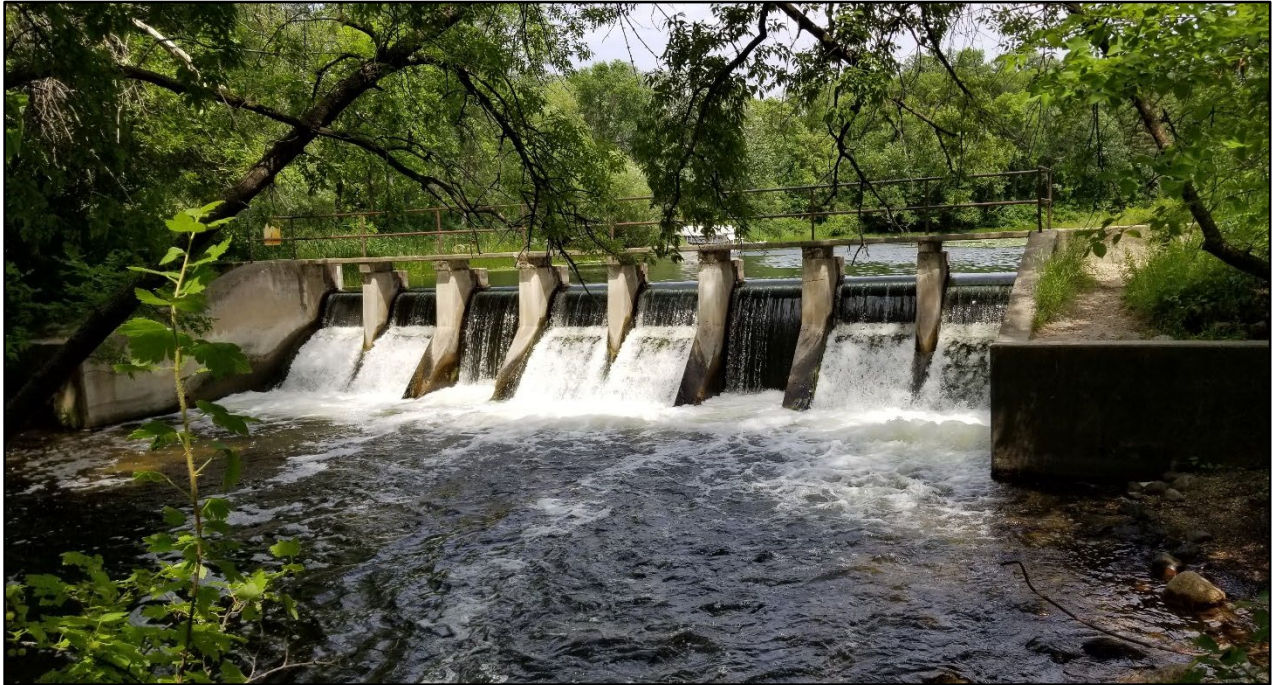
Photograph 2. Overview of Buck's Mill Dam, facing north/northeast (DNR 2020).
