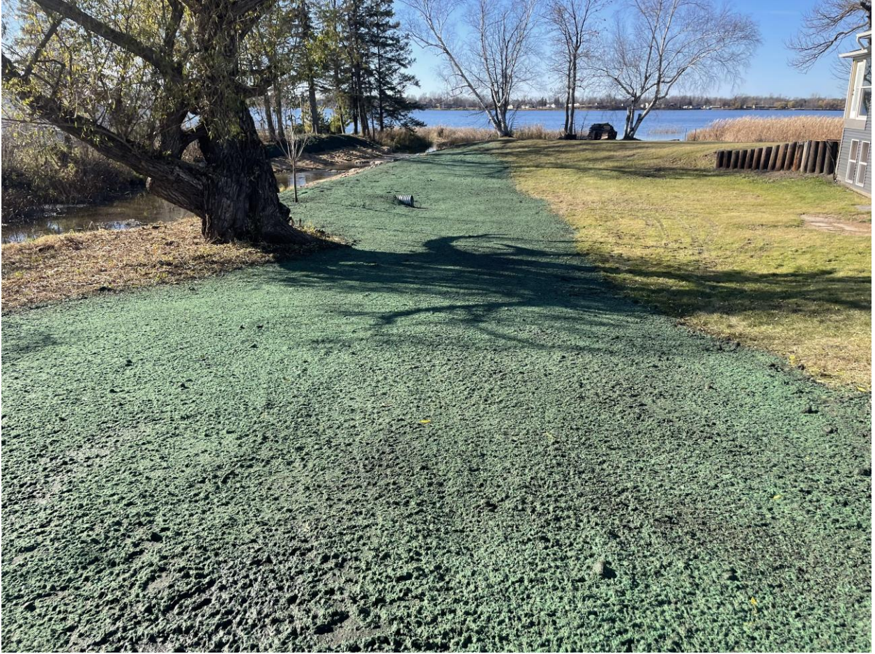
Seeding and hydro mulching over site finish grade.
