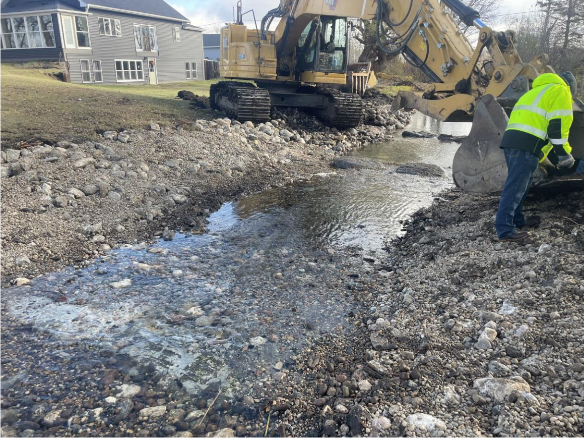
Weir installation throughout the rock arch rapids
