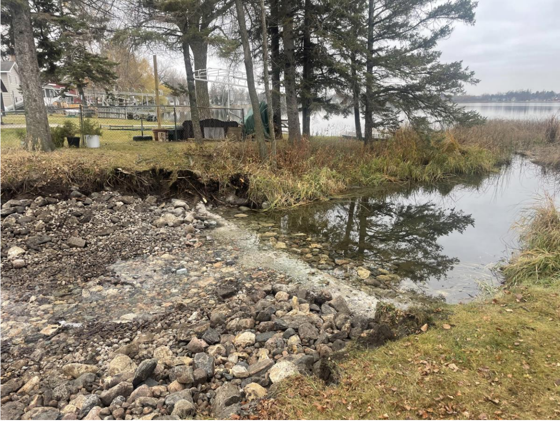
Modification of the existing dam
